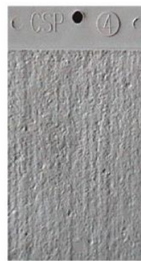
CSP-4: Light Scarification
