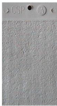
CSP-3: Light Shot Blast
